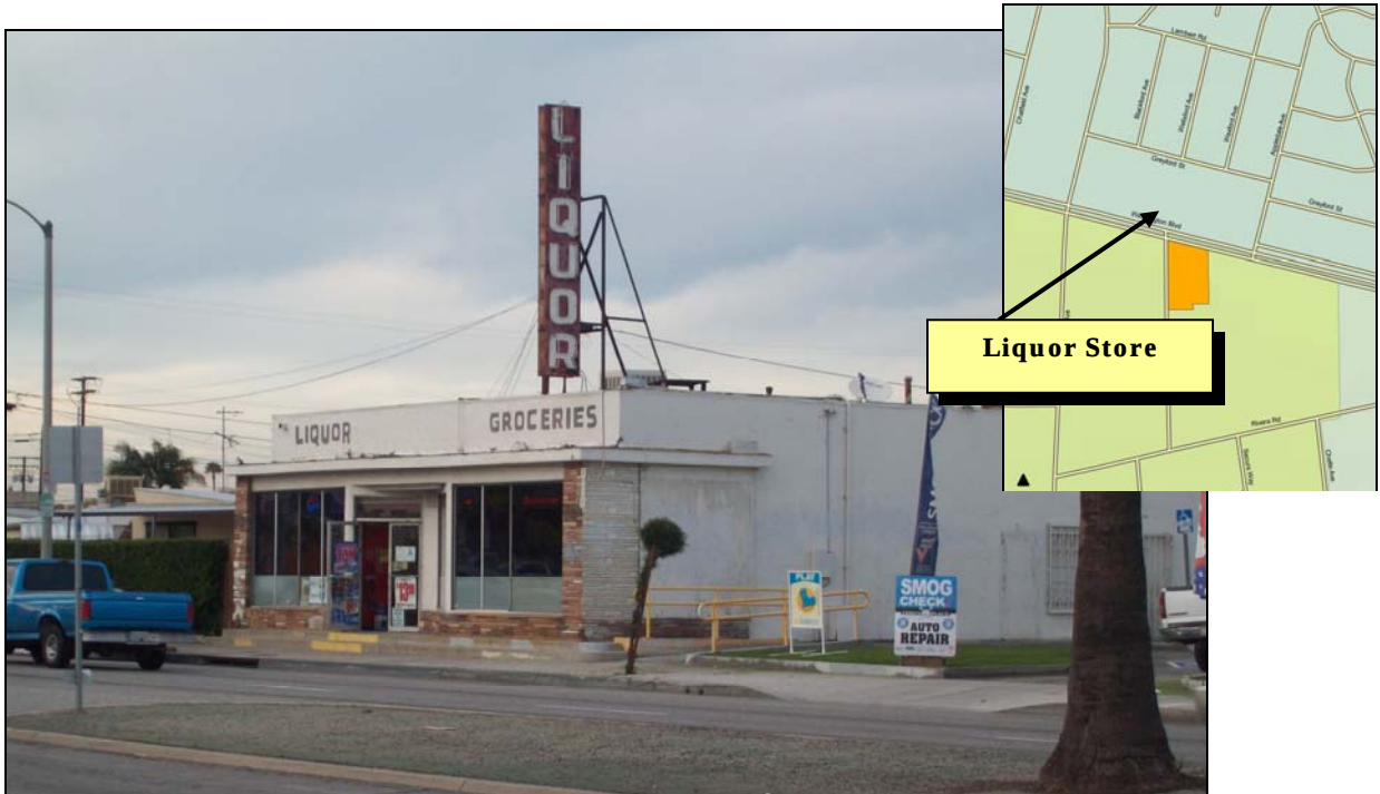
View of the liquor store facing northwest
