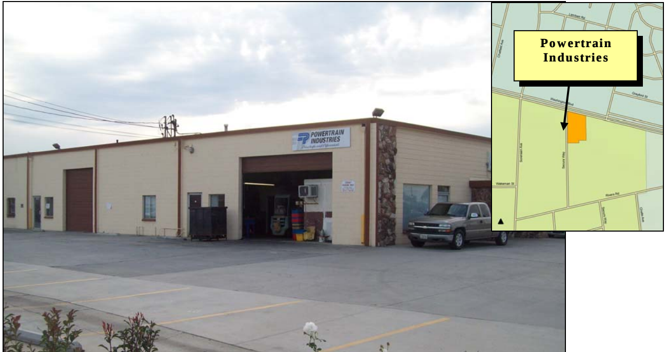
View of the Powertain Industries building located directly to the west of the project site
